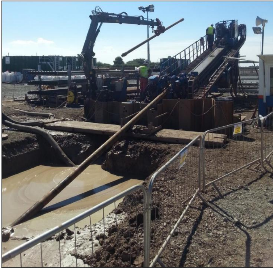
Figure 4.18: HDD rig carrying out landfall works at the Westernmost Rough offshore wind farm
